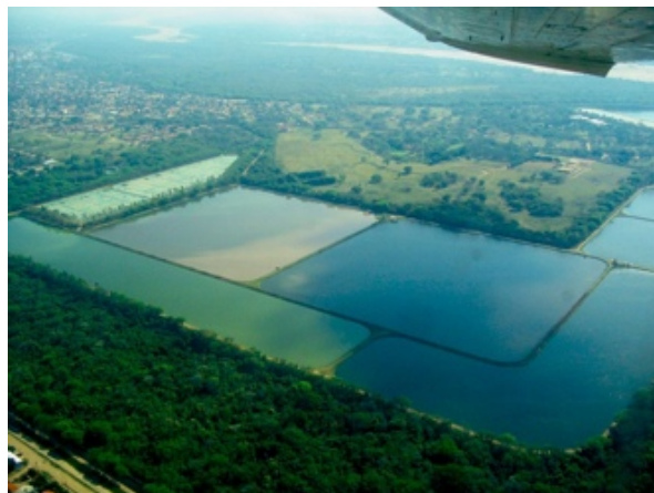
Pre-installation, the 2 primary lagoons can be identified by the poor colour due to oxygen deficiency.
