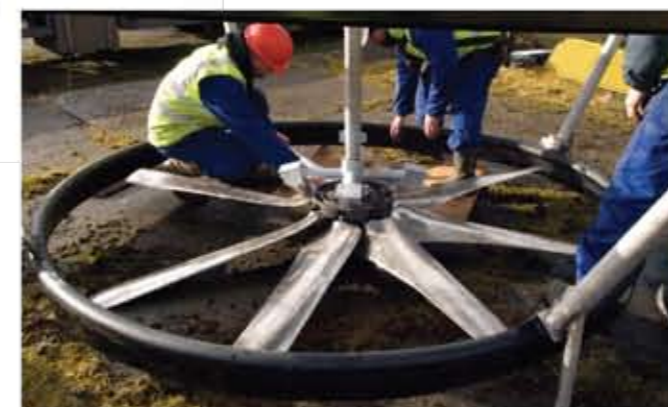
Above: Setting the pitch of the impeller to suit the reservoir depth. Right: Assembling the ResMix 3000 prior to installation
