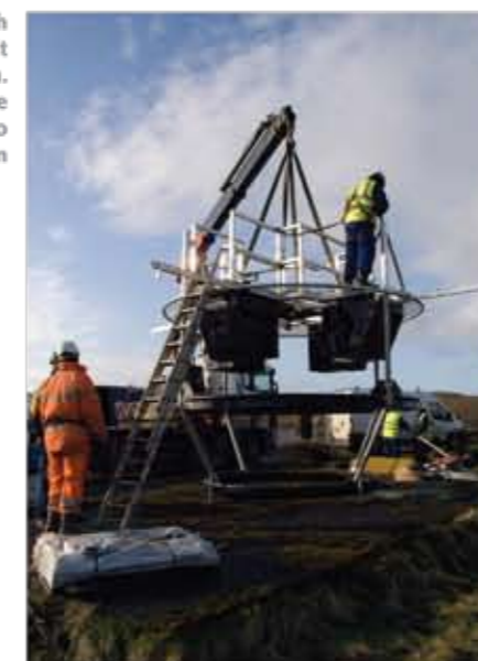
Above: Setting the pitch of the impeller to suit the reservoir depth. Right: Assembling the ResMix 3000 prior to installation
