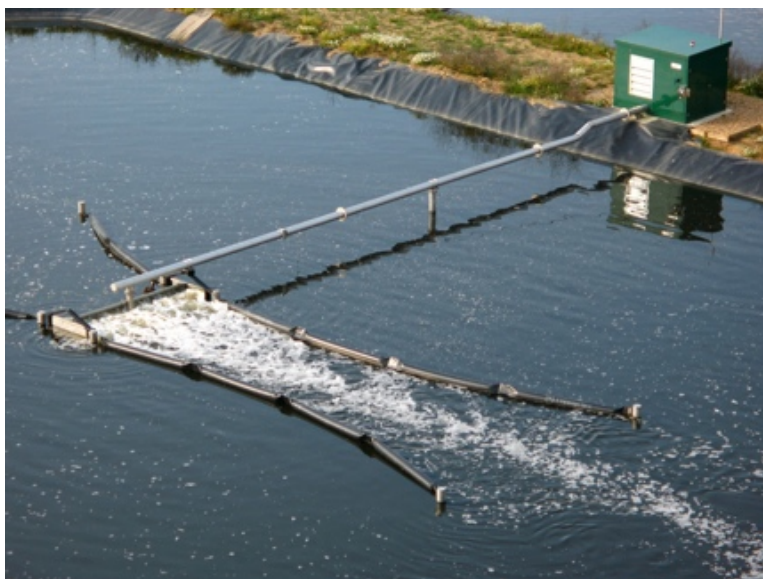
Photo 2 — The low maintenance Aero-Fac ® blower and diffused air aeration system.
